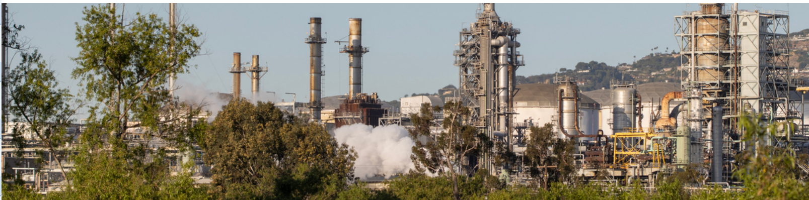
Exterior view of the Phillips 66 Los Angeles Refinery in Wilmington. Photo Credit: hapabapa
